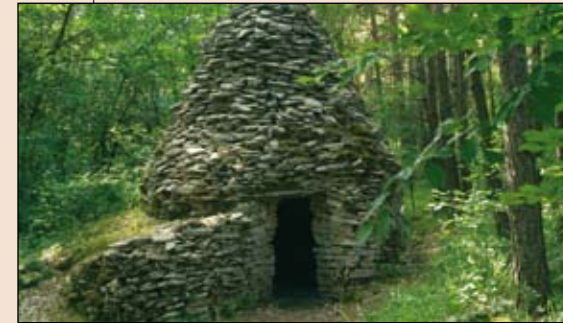
A cadole : a vine-grower's shelter made from dry stone.
