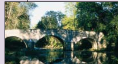
Stone bridge at Loches-sur-Ource.
